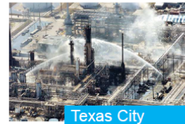
Texas City Refinery - 2005
