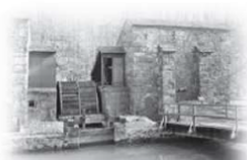
DuPont Black Powder Works in USA, 19tes Jhdt
